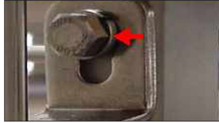
Figure 2. Principle 5: Hollow Areas Hermetically Sealed.
